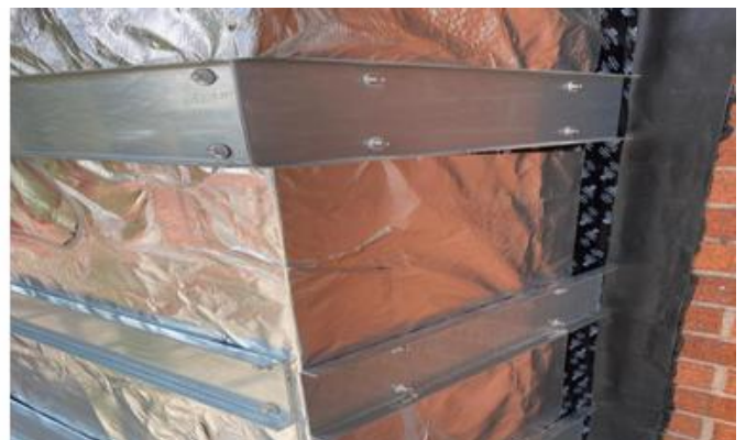
Progression on Elevation B
