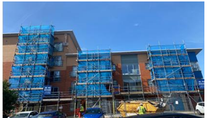
A photo showing scaffold complete and Membrane, and C channels being installed
