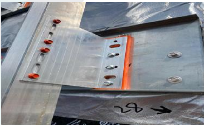
Progression on Elevation B
