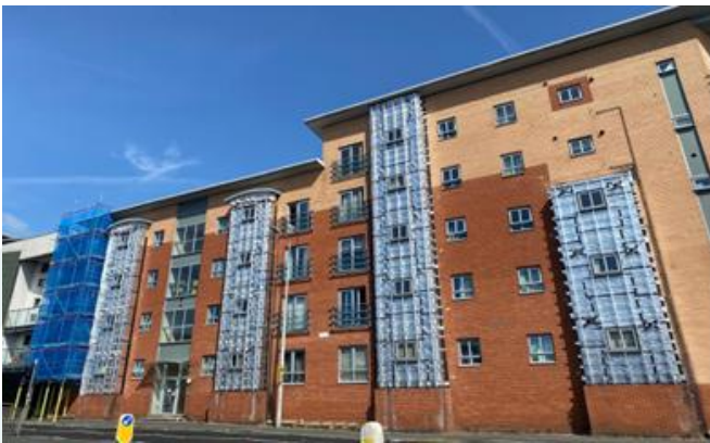
A photo showing Bracket and rails being installed
